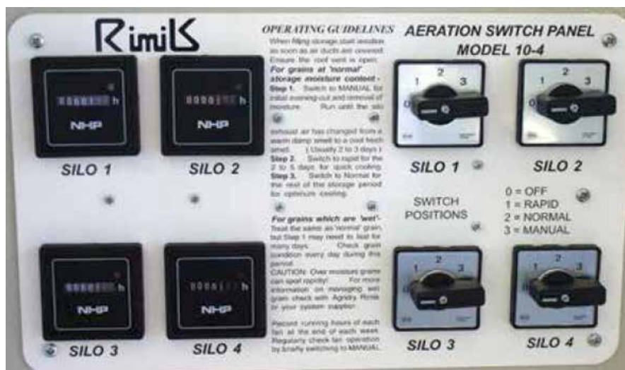
Photo 11: Automatic aeration controllers are the most effective way to cool grain and are designed to manage many storages, from one central control unit.
