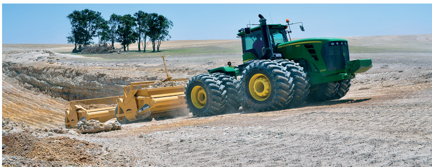
Spreading is more cost-effective when the clay pit is close to the area to be treated.
