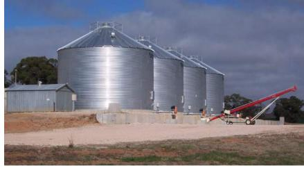
**Photo 3:** On-farm storage is becoming more sophisticated with aeration facilities and sealing capability to enable a quality product to be out-turned. (Photo: W. Hawthorne formerly Pulse Australia)
