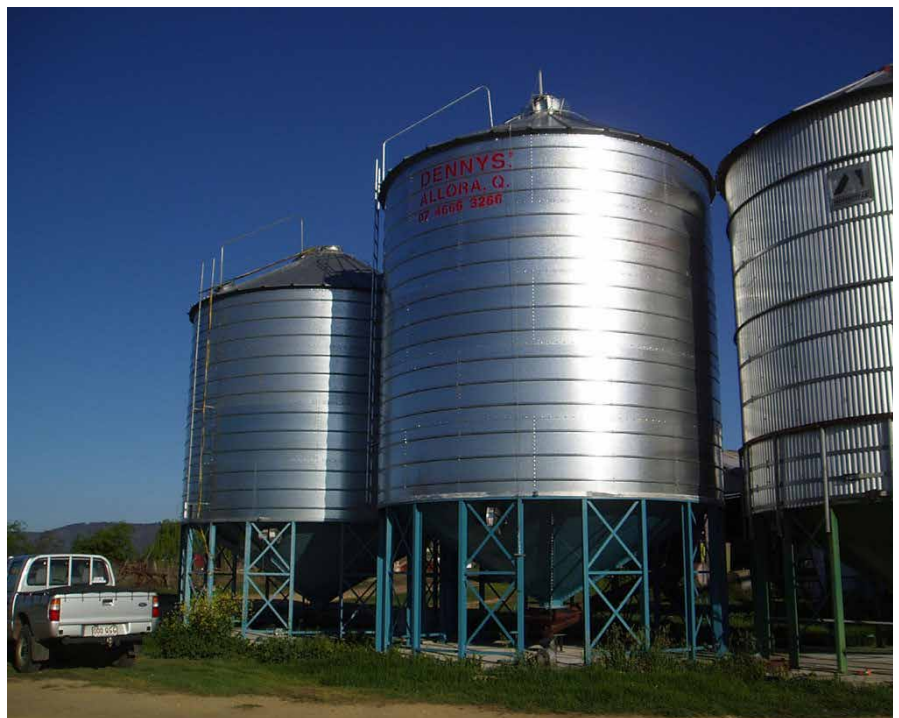
Figure 1: Aerated, sealable silo.
