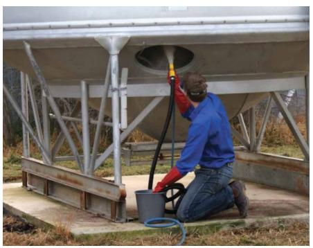
**Photo 8:** A blower and vacuum gun such as the Venturi gun is the best applicator for inert dusts. Aim for an even coat of diatomaceous earth across the roof, walls and base.
