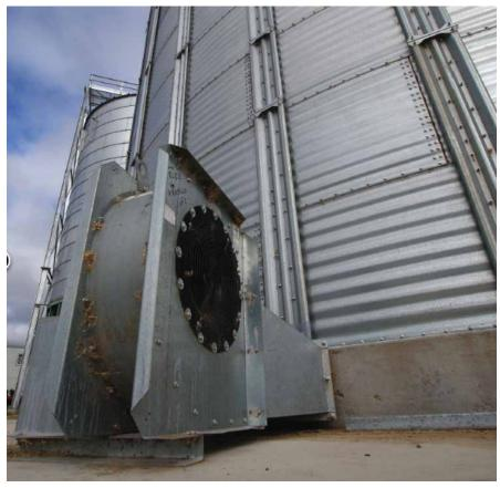
**Photo 10:** A flat-bottomed silo designed for aeration drying. Source: GRDC
