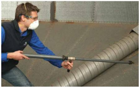
**Photo 6:** Clean silos, including the silo wall, with air or water to provide a residuefree surface to apply structural treatments. Source: GRDC
