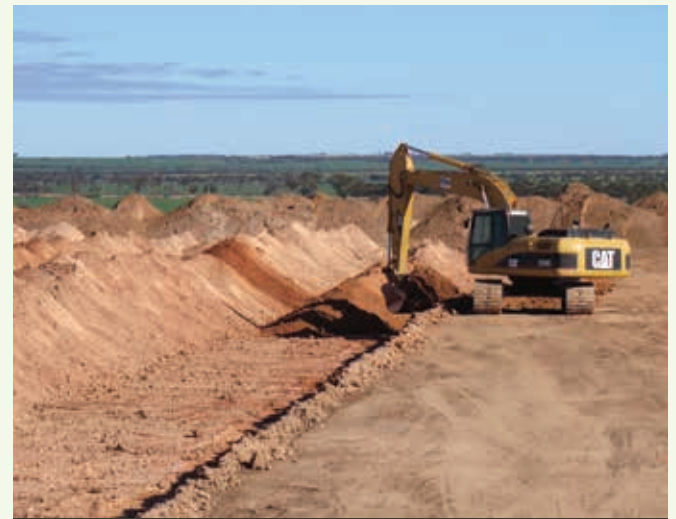
Stockpiling Morrel lime for the Nixon's 2016 liming program (Photo courtesy of Bob Nixon)
