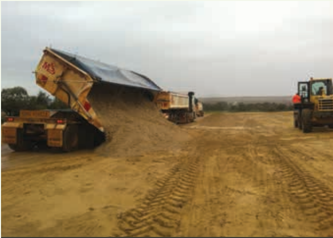
Another load of lime sand arrives for spreading. (Photos courtesy of Rod and Andrew Messina)
