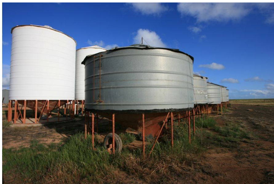
Photo 3: Silos painted white to reduce temperature.
