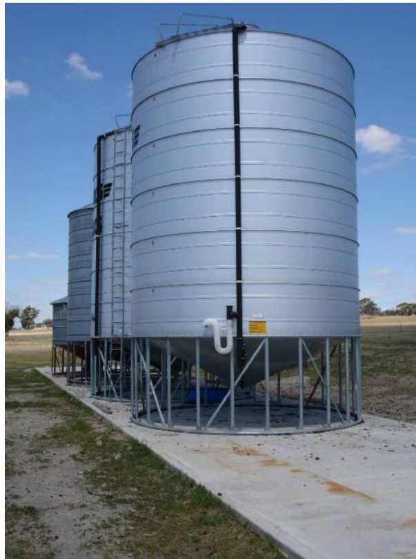
Photo 2: Sealable, aerated silos fitted with thermosiphons to assist with gas distribution during fumigation.
