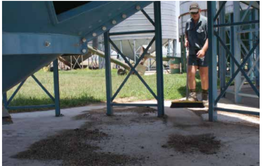
Photo 6: Concrete slab under silo makes cleaning up spilled grain much easier.
