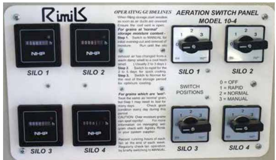
Photo 9: Automatic aeration controllers are the most effective way to cool grain and are designed to manage many storages, from one central control unit.
