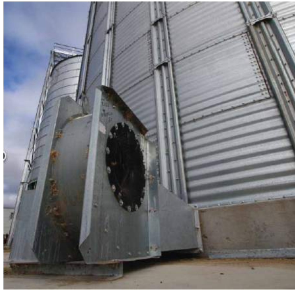
Photo 8: Aeration drying requires careful management, high airflow rates, well designed ducting, exhaust vents and warm, dry weather conditions.
