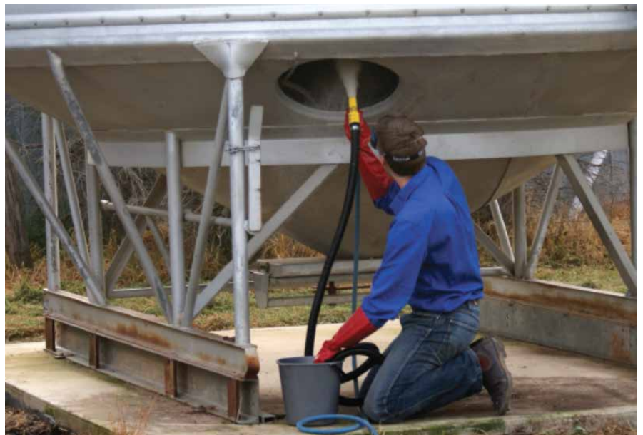
Photo 10: A blower/vacuum or Venturi gun are the best applicators for inert dusts. Aim for an event coat of diatomaceous earth across the roof, walls and base.
