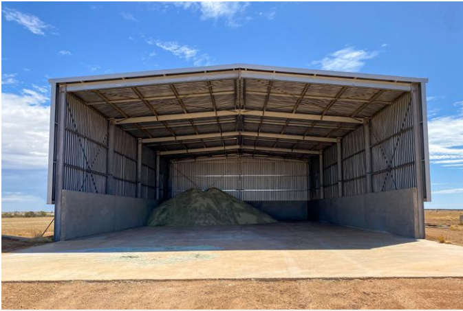
The original shed built in 2019 has 2.1m precast concrete walls and the back wall is 200mm thick to allow for additional pressure applied by the loader when unloading.
