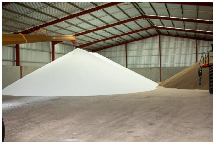
The slab of the multipurpose shed is 200mm thick and the tilt concrete walls are 2.7m high and are 170mm thick.
