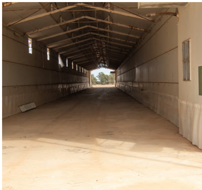
The chook shed was gutted and holes added along one side so fertiliser can be augered into the shed, which has the capacity to store 700t of urea and 1000t of MAP.
