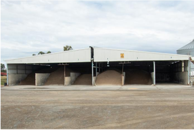
Roll-back roofs drive efficiency for unloading fertiliser and reloading grain at Godde's Grain & Fertiliser.
