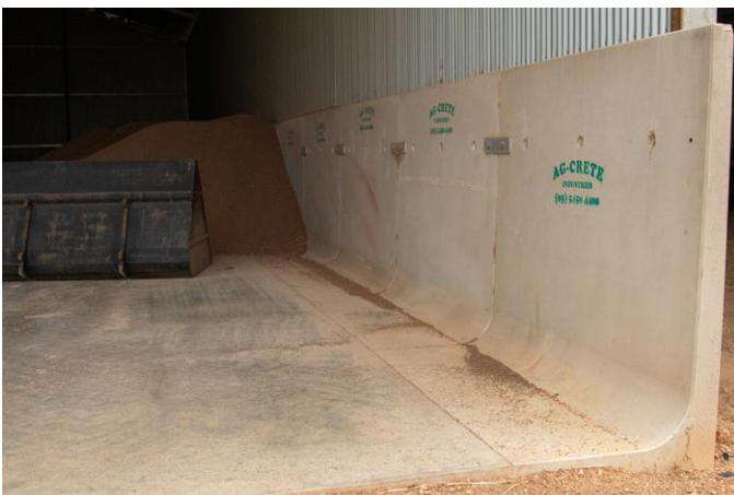
L-block (triangular) concrete wall system used in a bulk storage shed.
