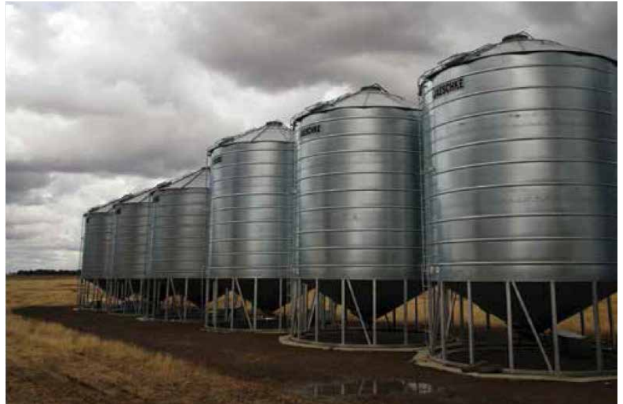
Photo 2: When using on-farm silos it is important to pressure test all silos, even those that are labeled as ‘sealed’.
