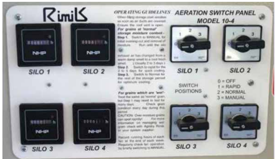
Photo 2: Automatic aeration controllers are the most effective way to cool grain and are designed to manage many storages from one central control unit.
