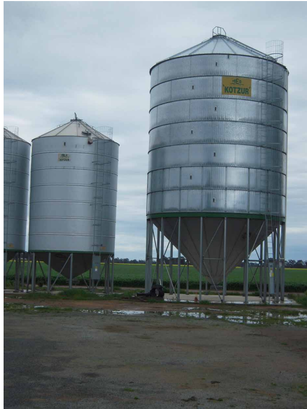
Photo 1: Storage silo with concrete slab underneath for easy cleaning.
