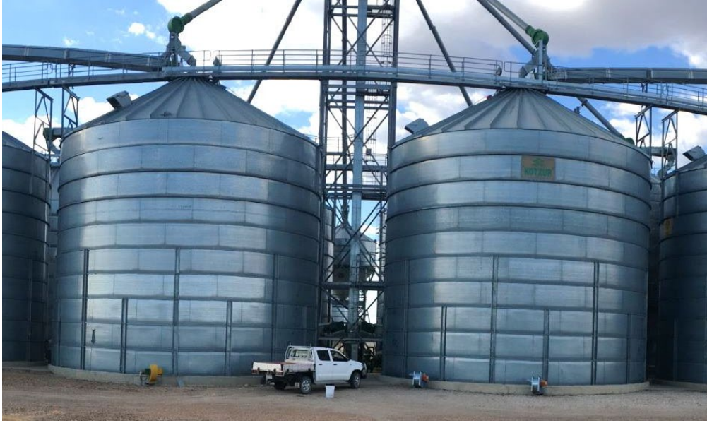
Figure 1. A farm storage facility with ten large flat-bottom silos, each with 1500 tonnes capacity (photo DAF Qld)
