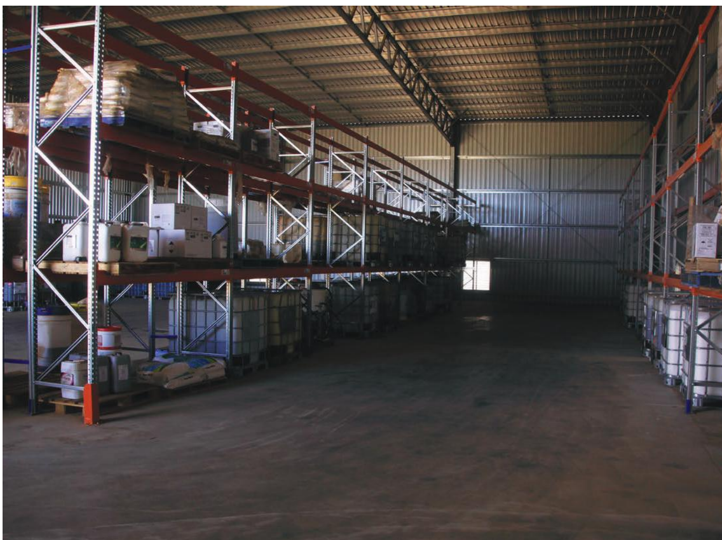
The chemical storage shed is fit for purpose – it keeps chemicals out of the weather and safely contained.
