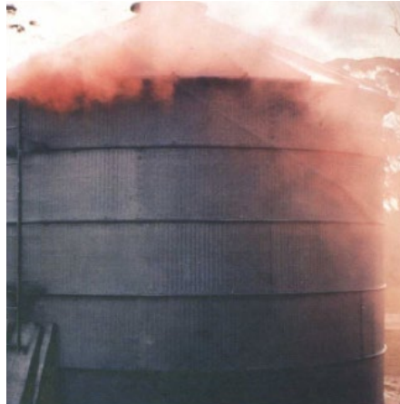
Photo 5: An unsealed silo.
