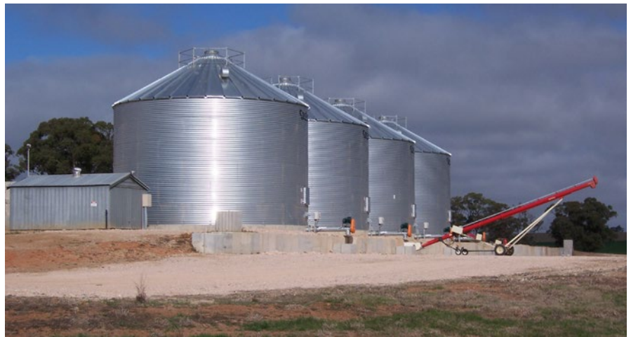
Photo 3: On-farm storage is becoming more sophisticated with aeration facilities and sealing capability to enable a quality product to be out-turned.
