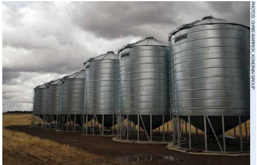
Photo 2: Sealable silos help growers protect triticale from insect attack, but for silos to remain effective, they must be maintained and regularly pressure-tested.
