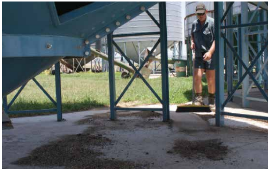
Photo 8: A concrete slab under silo makes cleaning up spilled grain much easier.
