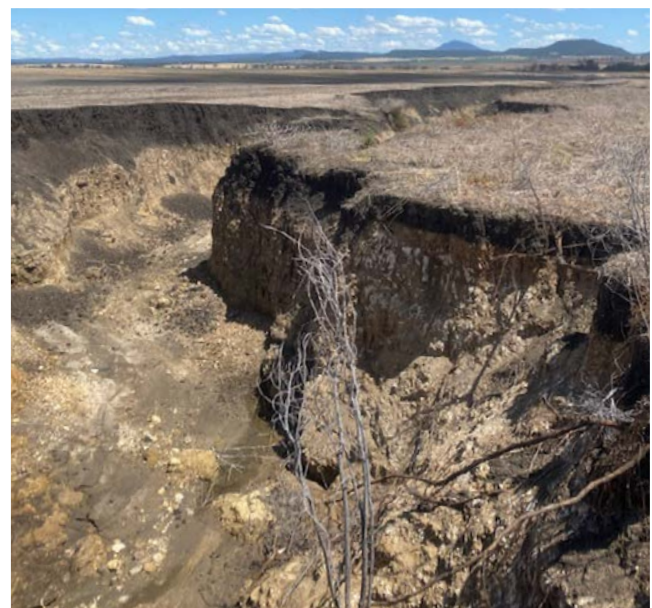
Erosion caused by back-to-back floods.
