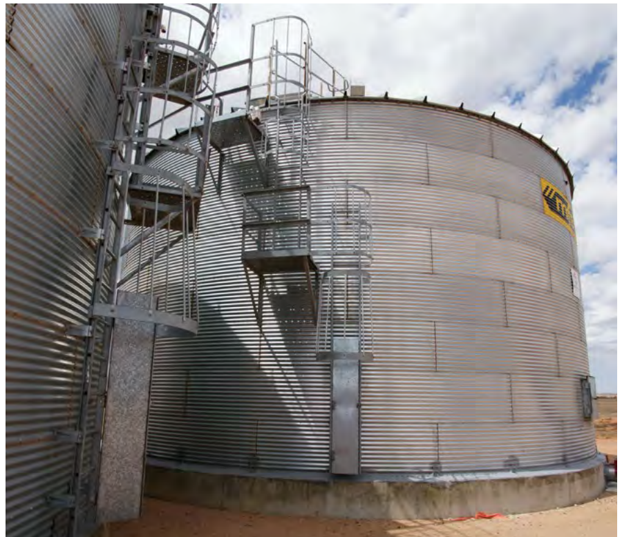
Photo 5: Caged and platformed access ladders improve safety when climbing the silo to inspect stored grain. (Source: Ben White, Kondinin Group)
