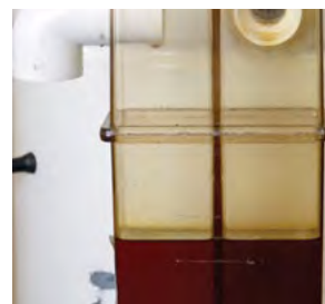
Photo 3: Ensure the pressure relief valve has enough oil to be level with the middle indicator mark. (Source: Chris Warrick, Primary Business)
