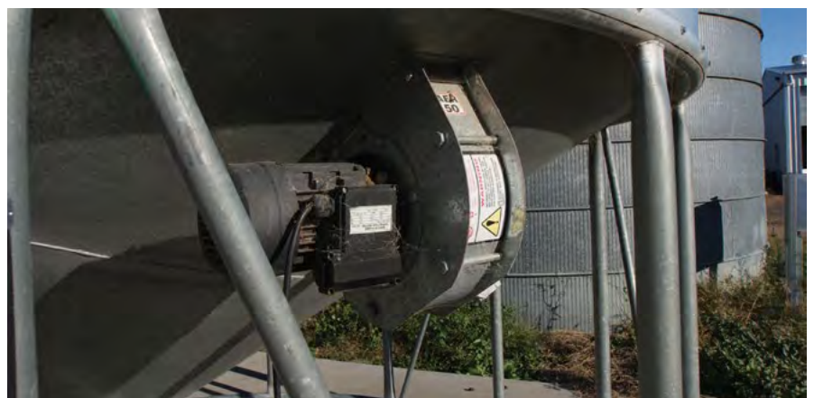
Photo 13: Aeration cooling is essential for storing oilseed and may require extra capacity to achieve 2–3L/s/t in small oilseeds such as canola. (Source: Chris Warrick, Primary Business)
