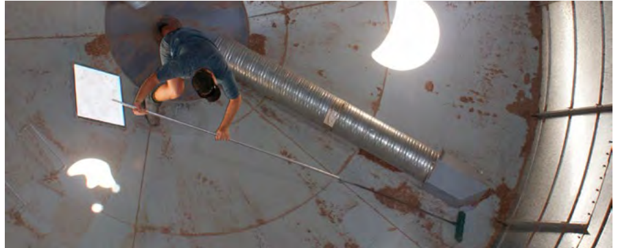
Photo 3: An extended broom handle makes sweeping out silos easier. (Source: Chris Warrick, Primary Business)
