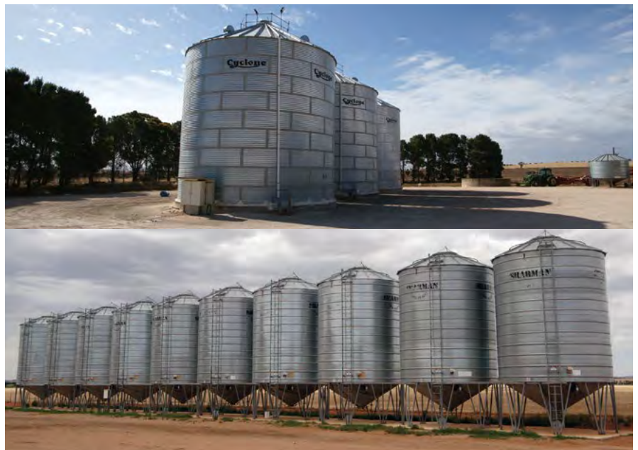
Photo 2: Flat-bottom silos (photo top) and cone-base silos (photo bottom) remain the most popular on-farm grain storage options. (Source: Chris Warrick, Primary Business)
