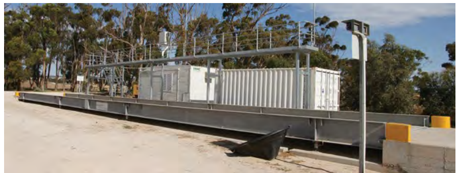
Photo 9: The addition of a weighbridge can help maximise truck carrying efficiency and avoiding overloading fines. (Source: Ben White, Kondinin Group)
