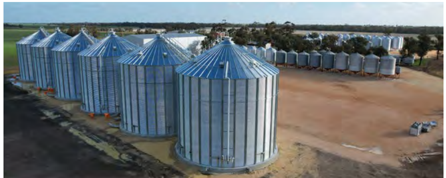
Photo 3: The choice between flat or cone-bottom silos requires consideration of ease of empty, segregation, efficient size for loading and unloading and cost. (Source: Chris Warrick, Primary Business)
