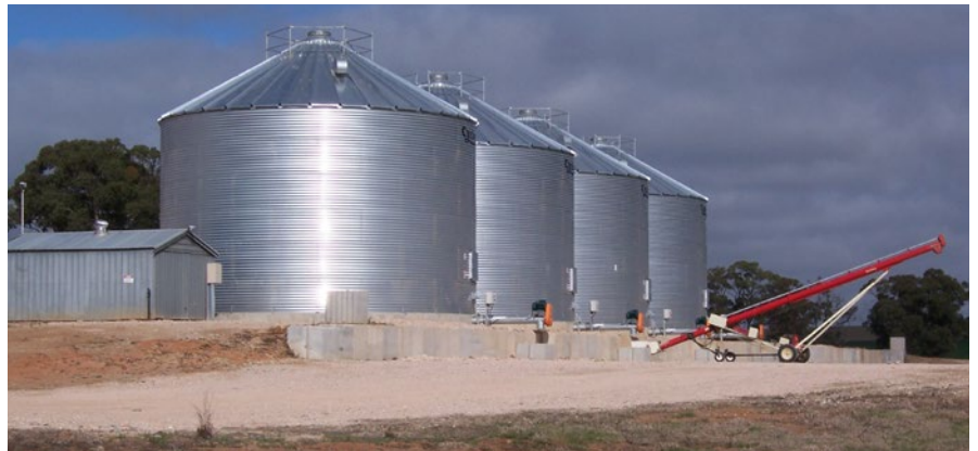
Photo 3: On-farm storage is becoming more sophisticated with aeration facilities and sealing capability to enable a quality product to be out-turned.
