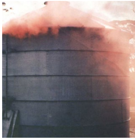
Photo 5: An unsealed silo.
