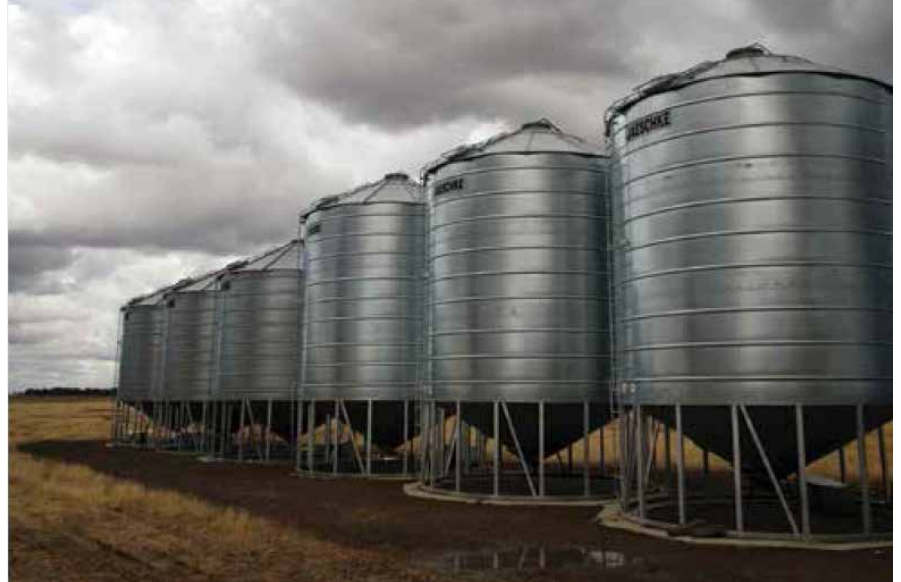
Photo 2: When using on-farm silos it is important to pressure test all silos, even those that are labeled as ‘sealed’.
