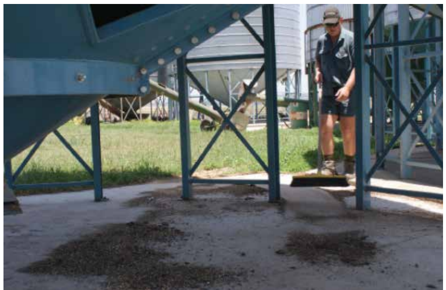
Photo 8: Concrete slab under silo makes cleaning up spilled grain much easier.
