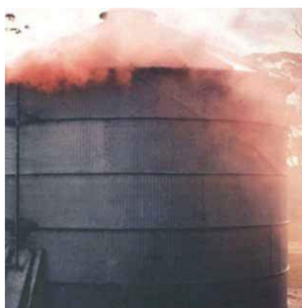
Photo 2: Using an unsealed silo for fumigation is both ineffective and dangerous.
