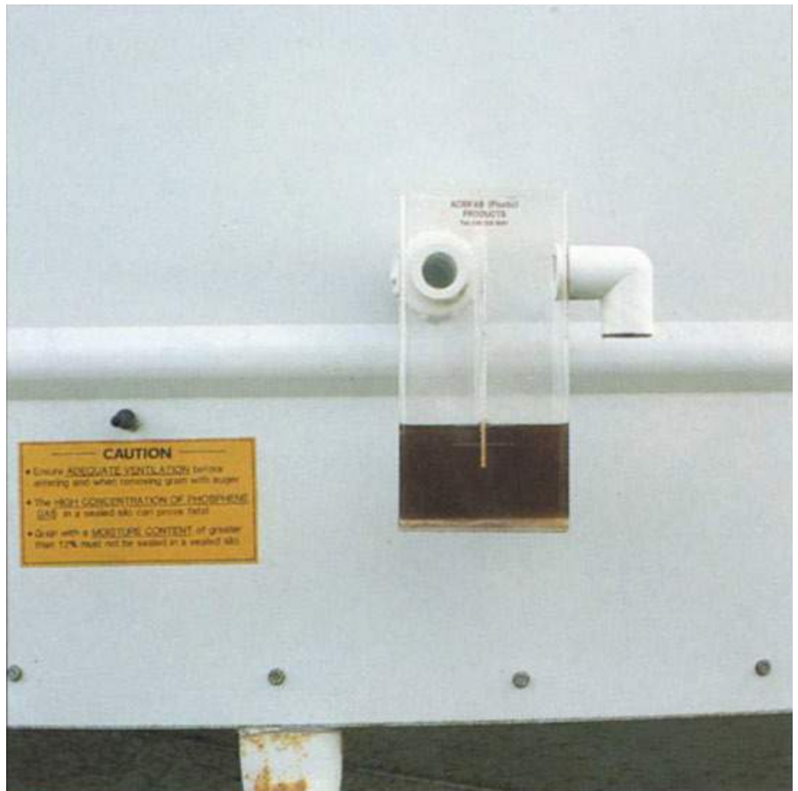
Photo 9: Pressure-relief valve on a sealable, gas-tight silo gives a quick means of checking the seal of the silo.
