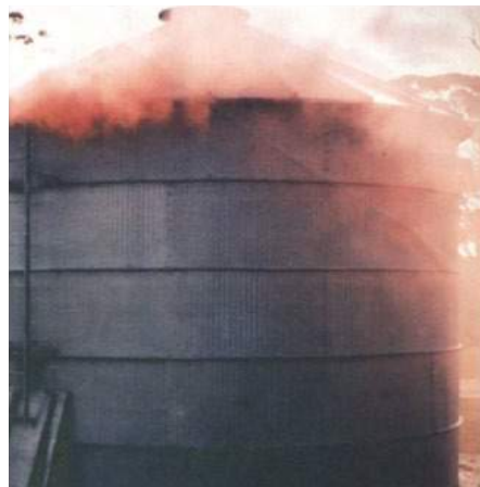
Photo 8: Unsealed silos are both ineffective and dangerous for fumigants such as phosphine.
