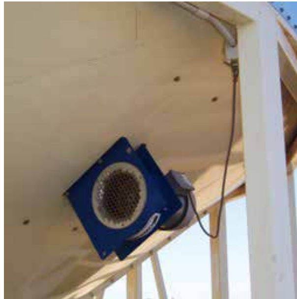
Figure 13: Standard aeration cooling fan. (Photo: Australian Oilseeds Federation)
