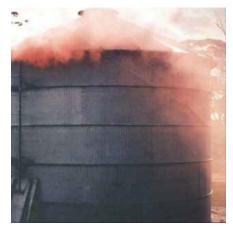
Photo 2: Using an unsealed silo for fumigation is both ineffective and dangerous. Photo: Grain Legume Handbook (2008)
