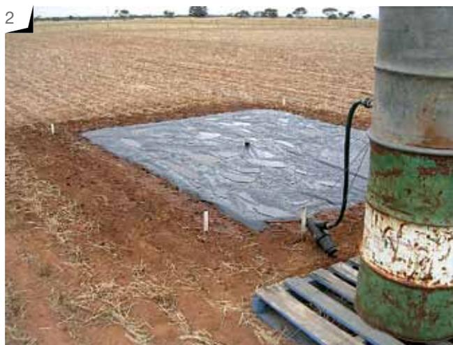
Photo 2: Completed pond showing header tank, in-line filter and wetted area covered in plastic sheet, the edges of which were placed in the trench before back filling with soil.
