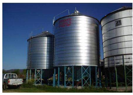
Figure 2: Aerated, sealable silos.
