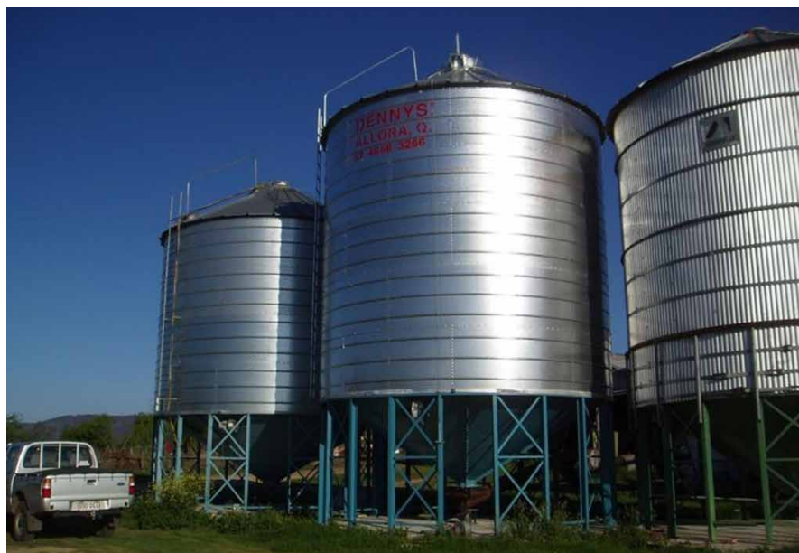
Figure 2: Aerated, sealable silos.
