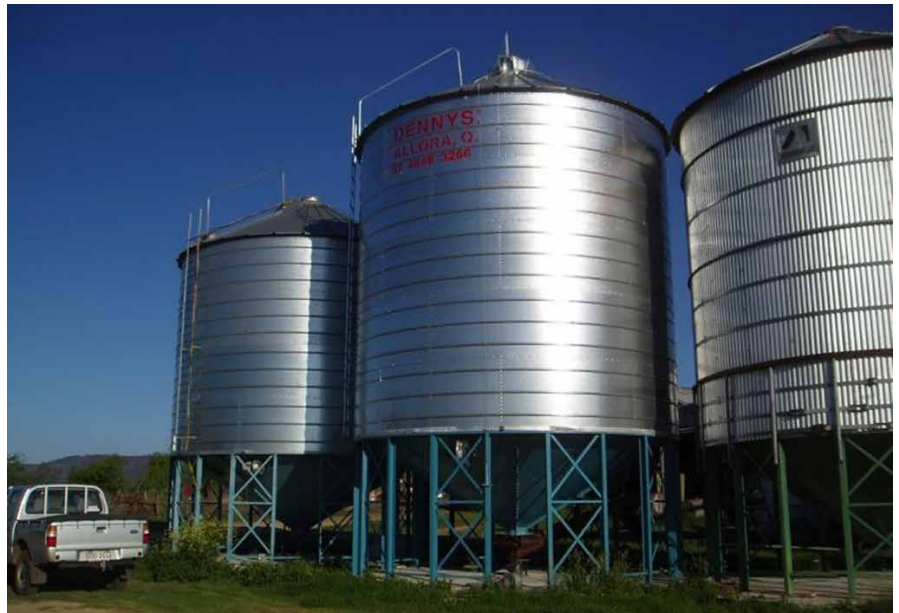
Figure 2: Aerated, sealable silos.
