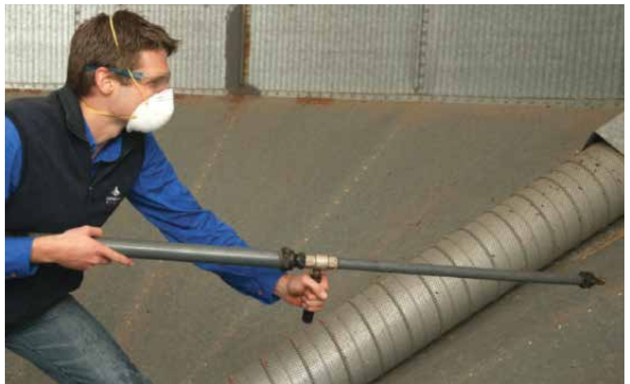
Photo 5: Clean silos, including the silo wall, with air and/or water to provide a residue-free surface to apply structural treatments.
