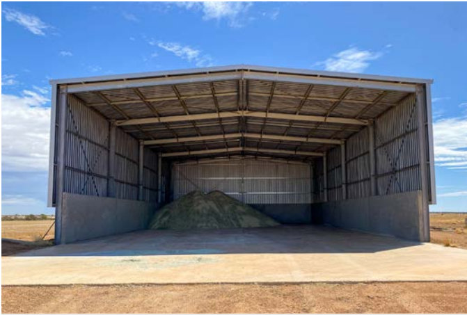
The original shed built in 2019 has 2.1m precast concrete walls and the back wall is 200mm thick to allow for additional pressure applied by the loader when unloading.
