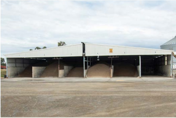
Roll-back roofs drive efficiency for unloading fertiliser and reloading grain at Godde's Grain & Fertiliser.
