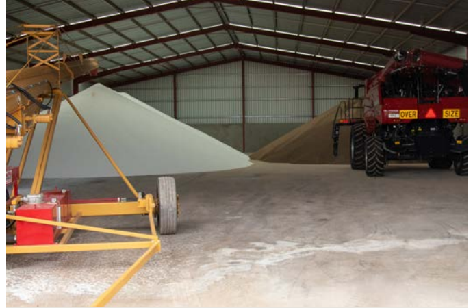
Shed height is important for the storage of machinery and for the ease of unloading fertiliser.
