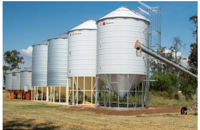
Purpose-built fertiliser storage silos, two silos on right, compared to grain silos.
