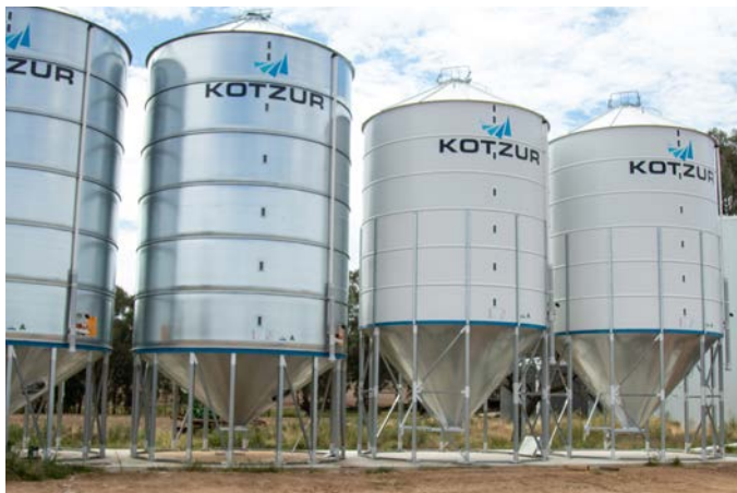
Fertiliser silos (right) have a steeper cone than grain silos (left).
