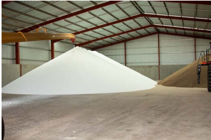
The slab of the multipurpose shed is 200mm thick and the tilt concrete walls are 2.7m high and are 170mm thick.
