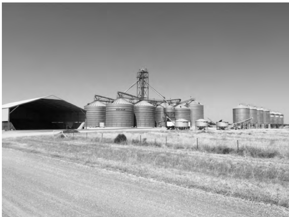
Figure 3. An on-farm storage facility with a weighbridge, sample stand and grain testing room.
