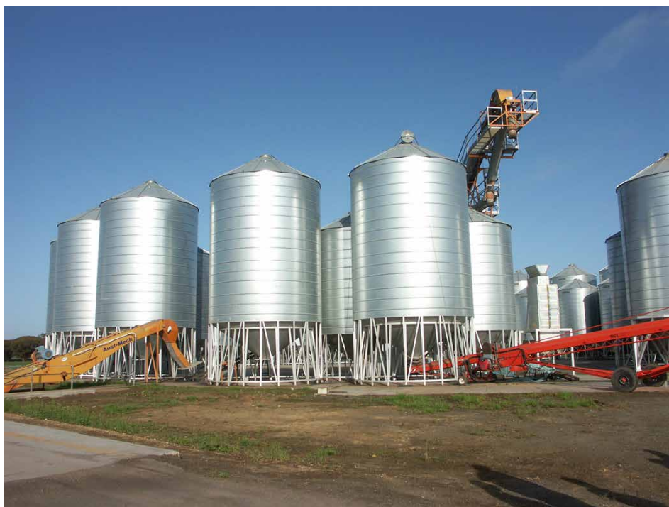
Figure 1: Meticulous hygiene and aeration cooling to manage storage temperature and moisture are crucial to prevent insect damage and moulds in stored chickpeas.
