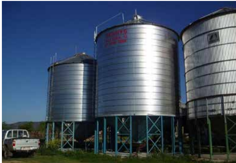
Figure 2: Aerated, sealable silos.
