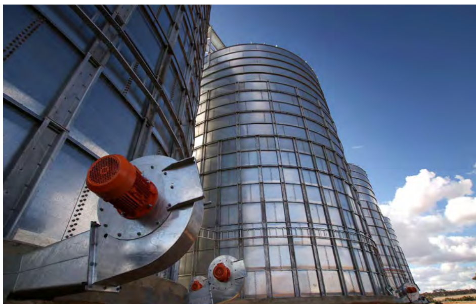
Figure 4: Aeration markedly reduces grain temperature. (Photo: Kondinin Group)
