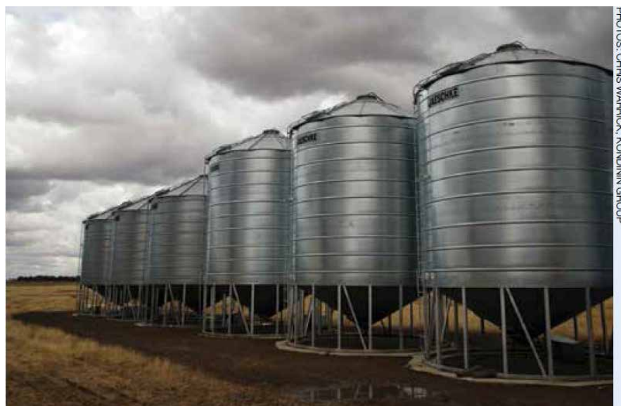
Photo 1: When using on-farm silos it is important to pressure test all silos, even those that are labeled as “sealed”.
