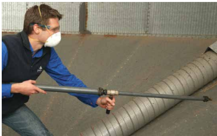
Photo 6: Clean silos, including the silo wall, with air or water to provide a residue-free surface to apply structural treatments.
