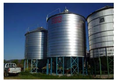
Figure 2: Aerated, sealable silos.
