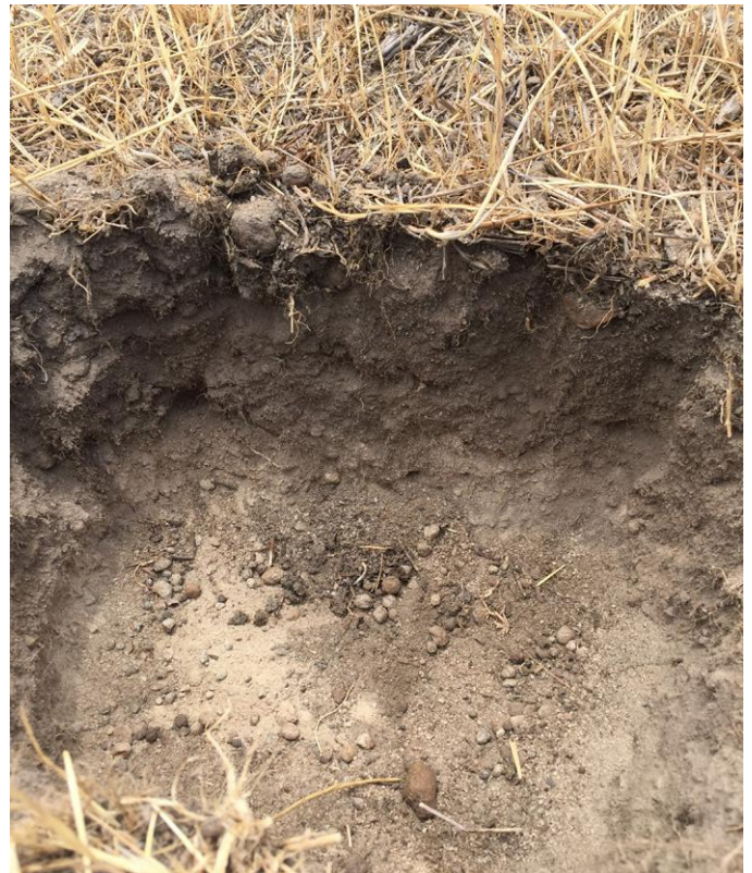
d) Gravelly sand (10 to 15cm) over dense next layer that is too hard to dig. pH testing required.
