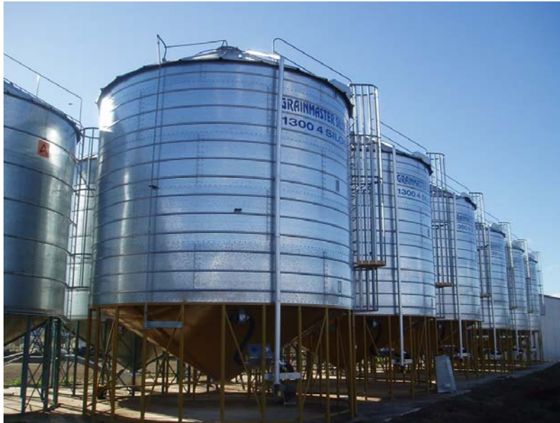
Figure 4. Silos fitted with aeration cooling and also designed to be sealable (air-tight) when required for effective fumigations
