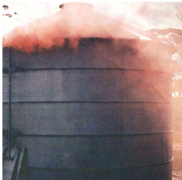
Figure 2: Obviously, this silo is not sealed. It is dangerous as well as ineffective with a fumigant such as phosphine.
