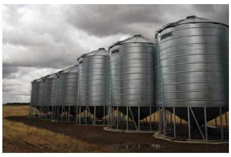
**Photo 2:** When using on-farm silos it is important to pressure test all silos, even those that are labelled as sealed.
