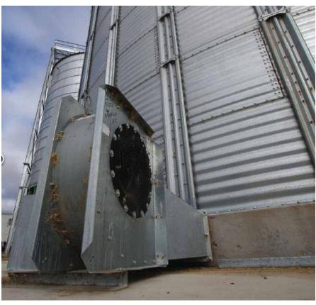
Photo 11: Aeration drying requires careful management, high airflow rates, well designed ducting, exhaust vents and warm, dry weather.
