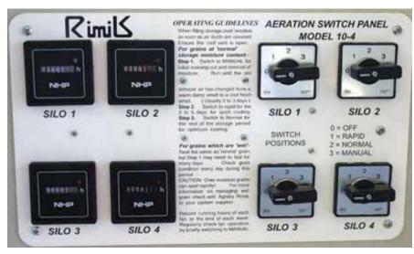
Photo 12: Automatic aeration controllers are the most effective way to cool grain and are designed to manage many storages from one central control unit.
