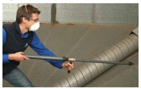
**Photo 7:** Clean silos, including the silo wall, with air or water to provide a residue-free surface to apply structural treatments.
